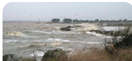
Storm surge topping levee at Hayward Regional Shoreline, 2005 Source: First Bay Regional Parks District
